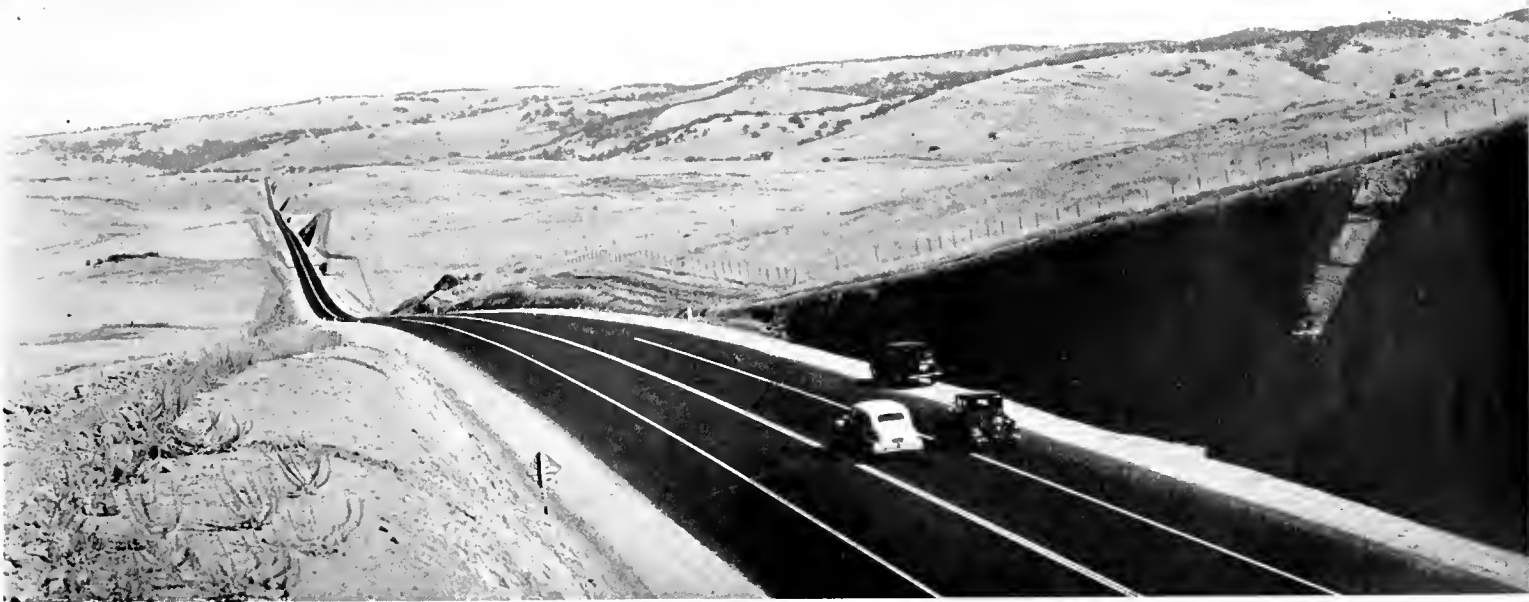
U. S. 50 realignment east of Folsom paved with plant-mix surfacing in 22- and 23-foot widths
